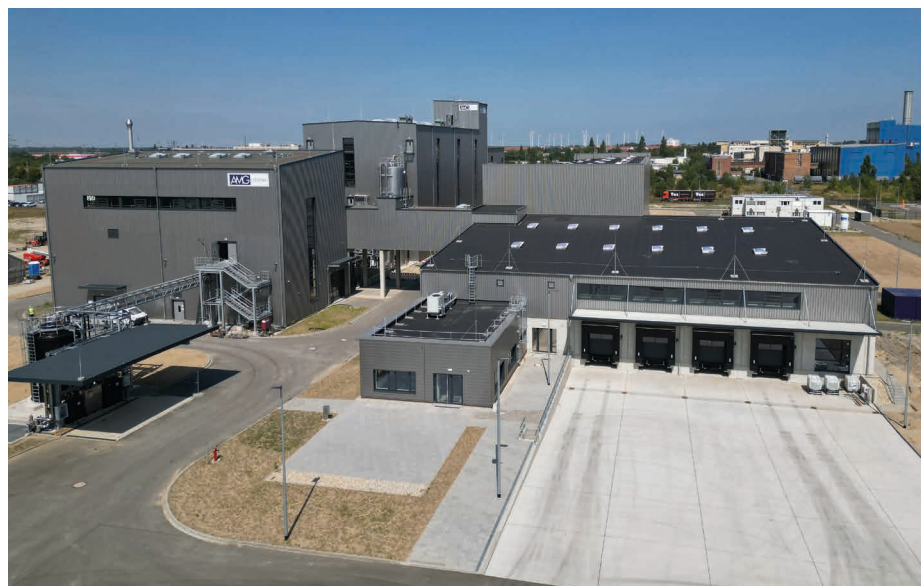
AMG Lithium GmbH's new lithium hydroxide plant in Bitterfeld-Wolfen, Germany.
